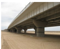
Awaza Bridge (TM)
