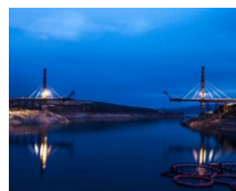
Agin Bridge (TR)
