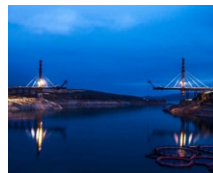
Agin Bridge (TR)
