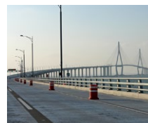
Incheon Grand Bridge (KR)
