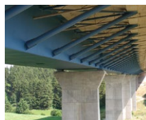
Steinbachtal Bridge (DE)
