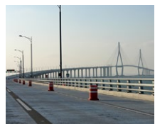
Incheon Grand Bridge (KR)
