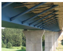
Steinbachtal Bridge (DE)
