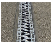
Cantilever finger joints
