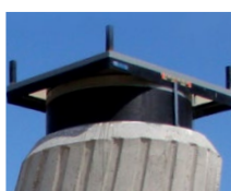
Deformation bearings
