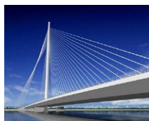
Tran Thi Ly Bridge (VN)
