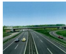
Freeway overpass Moosgasse, (CH)
