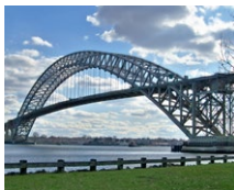
Bayonne Bridge (US)
