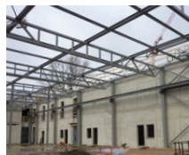
Factory building, Dusseldorf, DE
