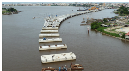
Approach span under construction
