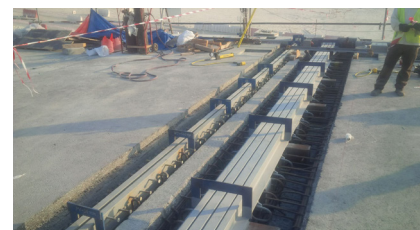
A TENSA®GRIP Type RS-B joint (on left) and a TENSA®MODULAR (LR3) joint before concreting
