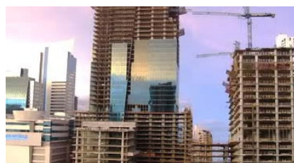
Construction of the Plaza
