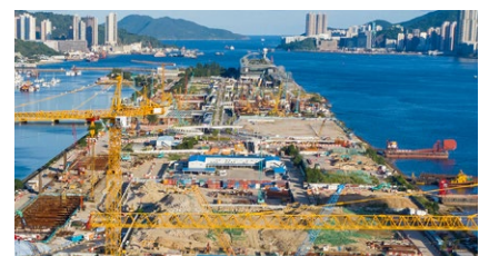
The Kai Tak Cruise Terminal during construction
