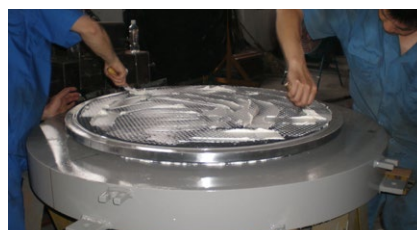
Application of grease to the upper sliding interface of a RESTON®SPHERICAL bearing
