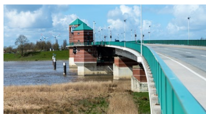
Approach to the Jann-Berghaus Bridge
