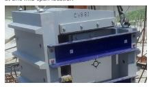
Following the installation of the hinge bearings, TENSA® MODULAR LR joints were installed
