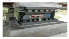
The installed spherical bearings are also equipped with dust skirts
