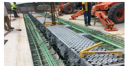
TENSA®MODULAR LR8-LS expansion joint equipped with noise reducing sinus plates
