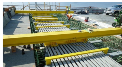
Installation of a 16-gap TENSA®MODULAR LR joint
