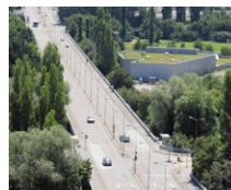
Europe Bridge (CH)
