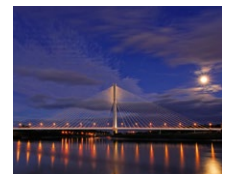
River Suir Bridge (IR)
