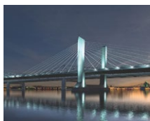
Ohio River Bridge (US)
