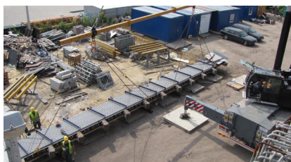
Preparation for lifting of a TENSA®MODULAR joint (type LR12) into position on the bridge
