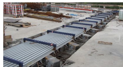
A TENSA®MODULAR joint of type LR12 during installation
