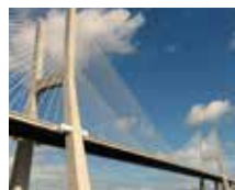
Vasco da Gama Bridge (PT)
