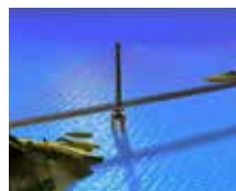
Agin Bridge (TR)
