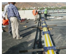
Fanja Bridge, Oman
