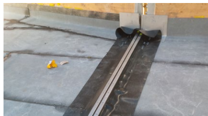
Le joint MIGUA installé
