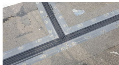
View of a mat joint TENSA®MAT with crossover
