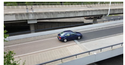
A car crossing the installed flexible plug joint POLYFLEX®ADVANCED PU
