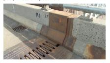
A TENSA<sup>®</sup>FINGER cantilever finger joint, as installed
