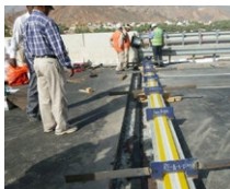
Fanja Bridge (Oman)
