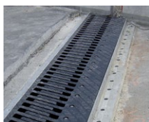
Sliding finger joints
