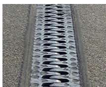
Cantilever finger joints
