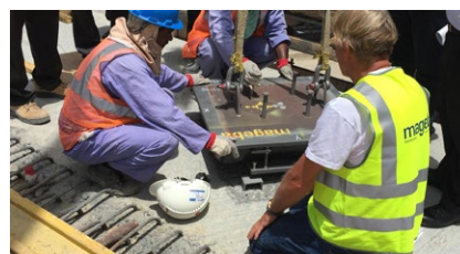
Lifting of a spherical bearing into its final position
