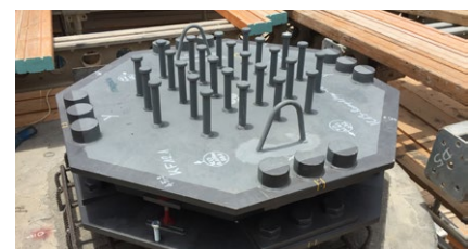
One of the installed RESTON®SPHERICAL bearings
