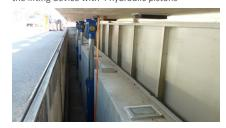
The sliding plate construction is fixed to the bridge
