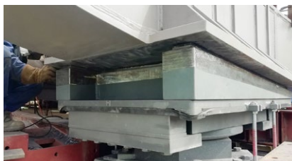
A RESTON®SPHERICAL bearing during installation
