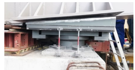
RESTON®SPHERICAL bearing in its final position
