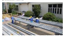
Installation of a large 24-gap TENSA®MODULAR LR joint
