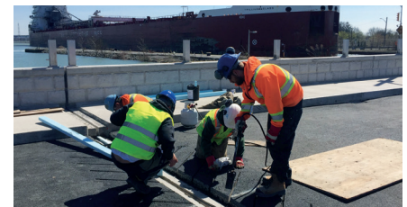
Installation of the POLYFLEX®ADVANCED PA30 expansion joint and support ribs
