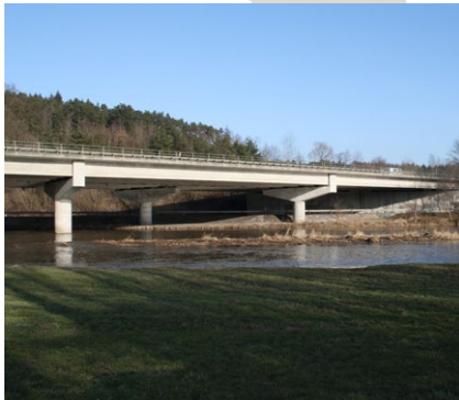
Naab Bridge | Germany
