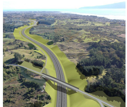
Mackays to Peka Peka Expressway | New Zealand
