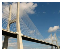
Vasco da Gama Bridge (PT)
