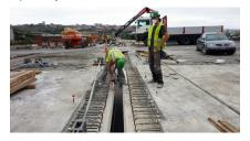
TENSA<sup>®</sup>FINGER expansion joints during installation on the bridge
