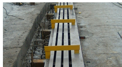
Installation of a TENSA®MODULAR expansion joint
