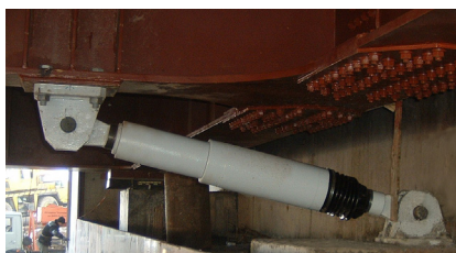
Installation of a RESTON®SA damper
