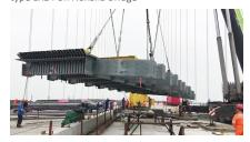
24-gap TENSA®MODULAR expansion joints were installed in the bridge's superstructure
