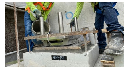
Grouting of a bearing plinth
