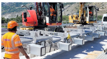
Lifting one of the TENSA®MODULAR LR-LS joints
