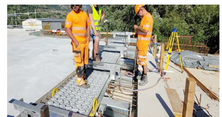
A type LR-LS modular expansion joint in its recess
