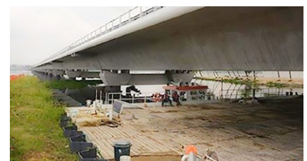
View of the bridge during construction
