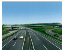
Freeway overpass Moosgasse, (CH)
