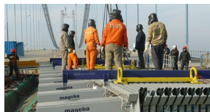
An 18-gap TENSA®MODULAR LR expansion joint is ready for installation
