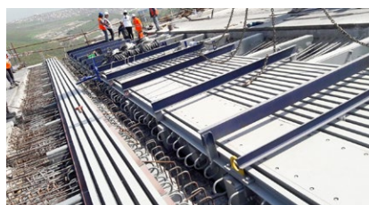
Installation of an expansion joint with fuse element
