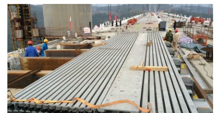
Installation of the joints with the patented fuse system element
