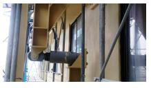
All 296 RESTON®SA dampers were successfully tested before installation
