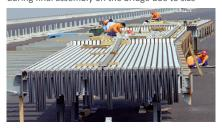
View of the underside of a TENSA®MODULAR joint of type LR27, prior to installation
