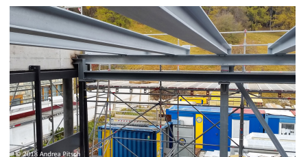
The bridge crane's steelwork support structure during construction
