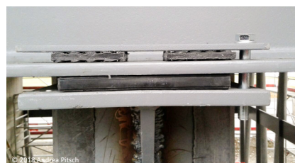
Elastomeric bearings during installation on support bracket
