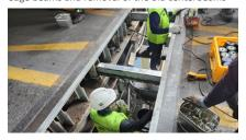
New centerbeams are being installed and connected to the support bars beneath
