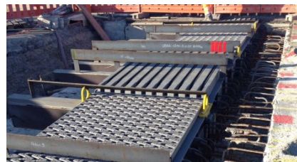
TENSA®MODULAR SILENT expansion joints of type LR10-LS100 with detail for the central reservation
