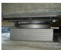
Spherical bearings
