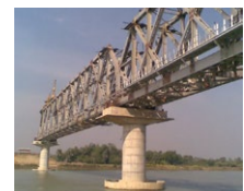
Bhagirathi Rail Bridge (IN)
