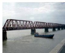
Bhairab Rail Bridge (BD)
