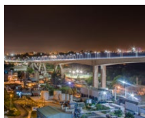
Chilina Bridge (PE)
