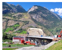
A9 motorway – Raron (CH)
