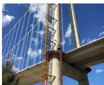
Longjiang Bridge (CN)
