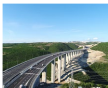
Liman Viaduct (TR)
